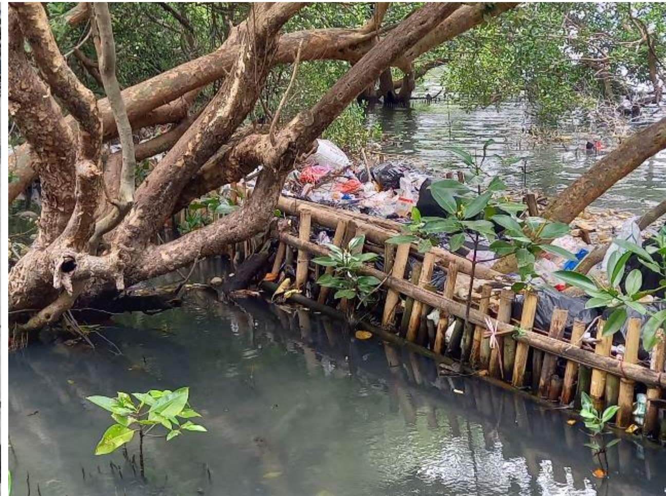
↑ Bamboo fence to prevent marine plastics entering mangrove forest in Jakarta Bay, Indonesia. November 2022, Indonesia, photo by M. Kojima.
