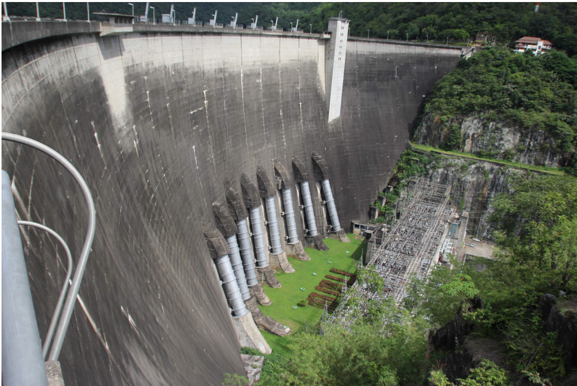
Photo: Phumiphon Dam from the crest. Eight outlets from the dam body (center) connected to the power house (bottom right) are seen (September 22, 2012 by the author)
