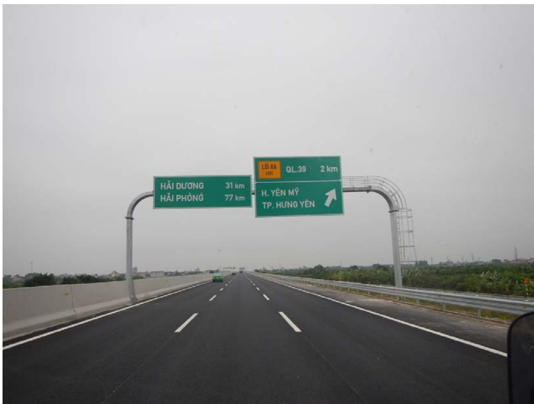
Figure 6.1. Example of Road Signs on the Hanoi–Hai Phong Expressway
