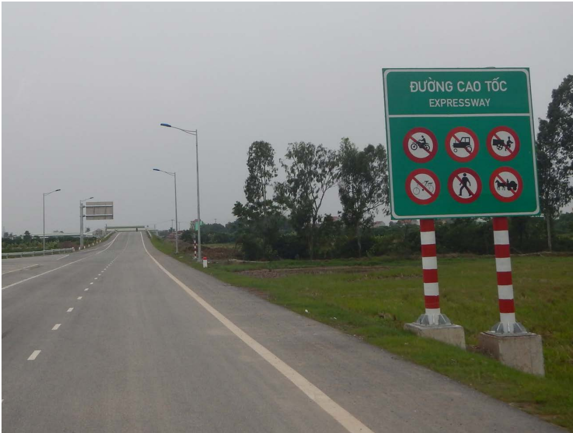
Figure 6.2. Example of a Road Sign at the Entrance of the Hanoi–Hai Phong Expressway
