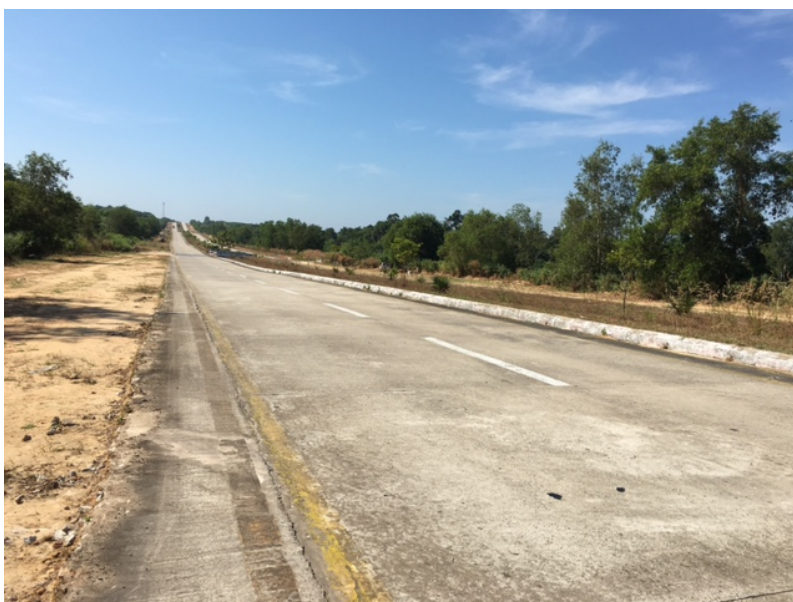
Figure 5.6. Section of the Yangon–Mandalay Expressway
