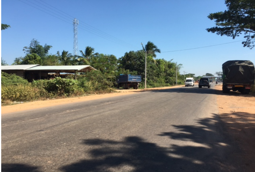
Figure 5.8. Road Conditions at the Phayagyi–Myawaddy Section of AH1
