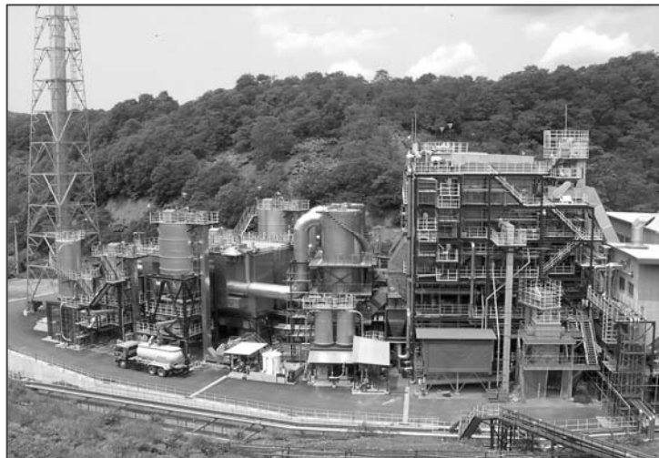
Incinerator for auto shredded residue using the copper smelter infrastructure. Provided by Kosaka Smelting & Refining Co., Ltd.
